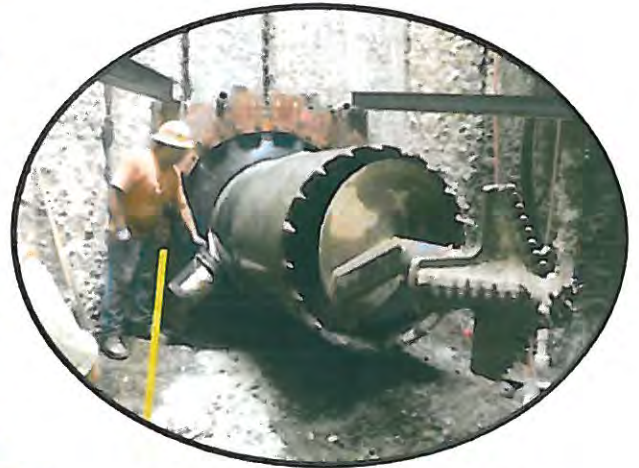
Trenchless - Casing Entering Shaft 6
