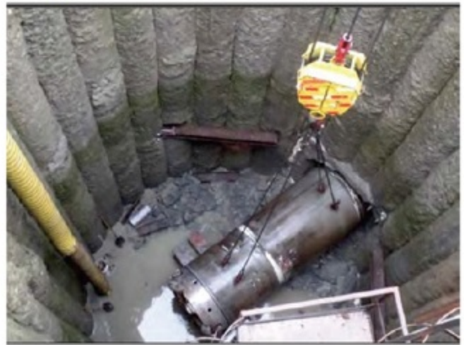
Trenchless—Tunneling Machine Entering Shaft 3
