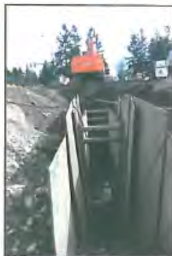
Construction at Covington Way SE & 168th PL SE
